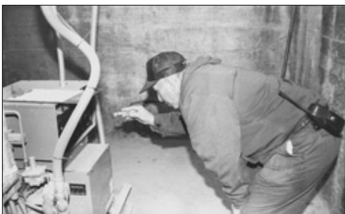
Kevin Claussen, maintenance, leans over and checks the readings on the back-up generator located in the student center. Claussen is in charge of the heating and air conditioning on campus. The back-up generator is tested during the weekend to make sure it is always in working condition. His job also demands that he checks five boilers that provide heat for campus. All five are checked daily to make sure they are in working order.
